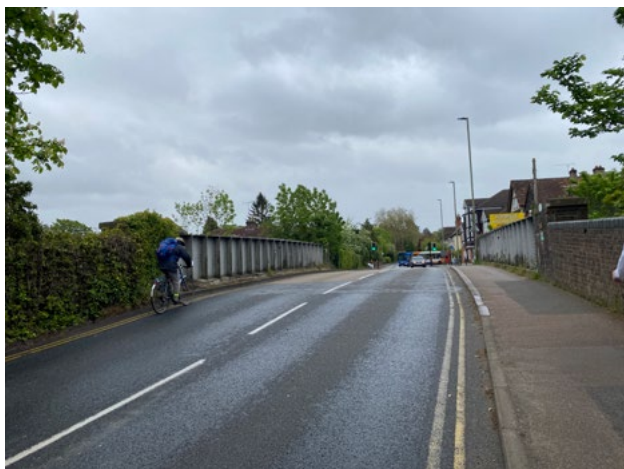
Figure 69. Missing footway on the bridge above the railway lines
