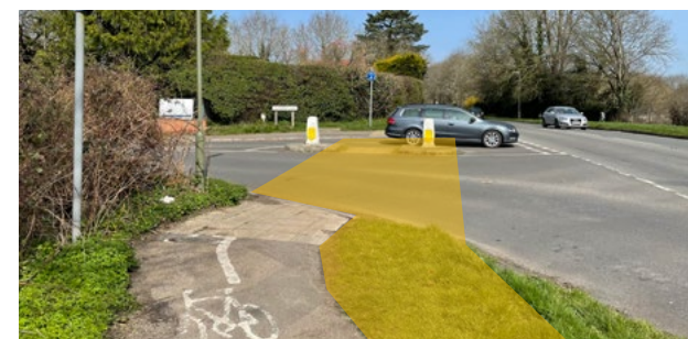
Figure 46. Weybourne Road at Monkton Lane - proposed path widening to provide segregated two-way cycle track and footway, and raised table for cycle priority at side road junctions (proposal #2; highlighted in orange) [source: Google Streetview]
